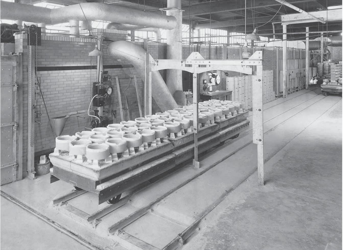
The gas-fired tunnel kiln greatly increased the quality and quantity of fired ware. The loading of the small cars was crucial, the ware had to be stacked carefully, so that it received the heat evenly and did not collapse. A kiln wreck could result if a stack collapsed, requiring the kiln to be completely shut down, a process that took several days. **The Akron Porcelain & Plastics Co.**
